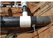
Kebu Rockshield PP 500 is used as additional mechanical protection for coatings in accordance with DIN 30672 and DIN EN 12068 as well as for buried plastic, steel and cast iron pipes and containers. Depending on the nature of the soil, it also makes it possible to partially or completely dispense with sanding. It has a shock-absorbing and load-distributing effect.
